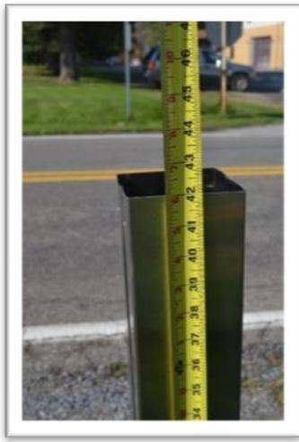
Using the measuring tape, measure 41 inches up from the ground level to the top of the post to ensure that it will be 41 inches off the ground once the concrete has cured.
