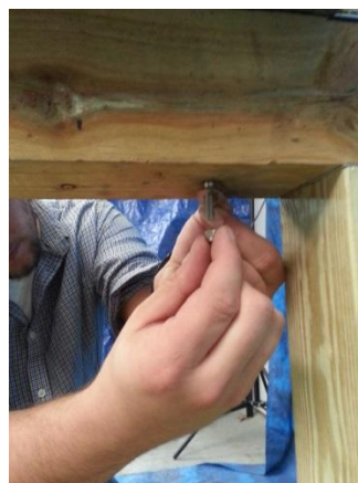
WHILE YOU THREAD THE WASHERS AND LOCK NUTS ON THE END OF THE BOLTS
